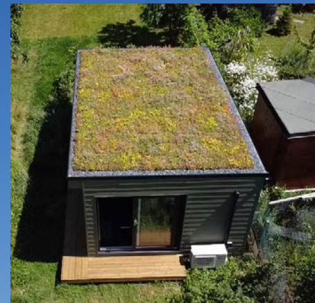
Green sedum roof
